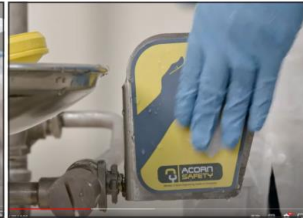
How to use the eye wash station push down the lever shot
