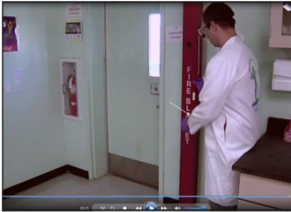
How to use the fire blanket Location of fire blanket
