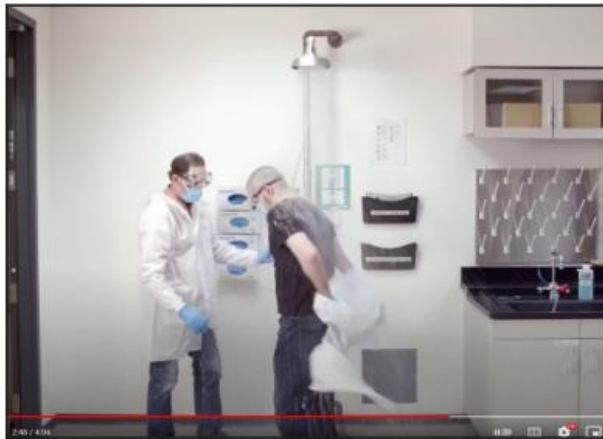
How to use the safety shower. Taking off cloth while washing, full shot
